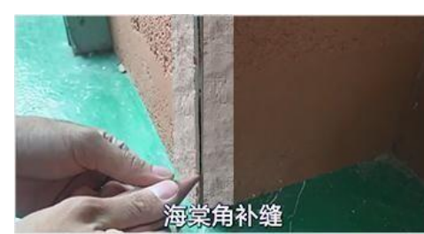
8. Fill the external corners with caulk
