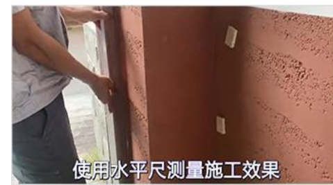
4. Measure the construction size with a ruler
