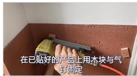
3. Fit it with air nails
