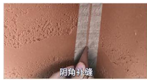
7. Fill the internal corners with caulk
