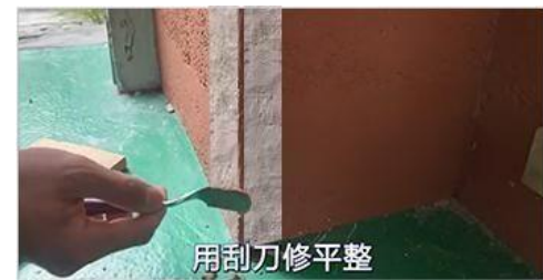
9. Use a scraper to smooth the caulk
