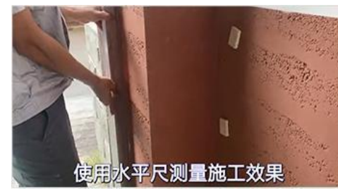
3. Measure the construction size with a ruler
