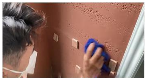
5. Clean it with a dry cloth after paving
