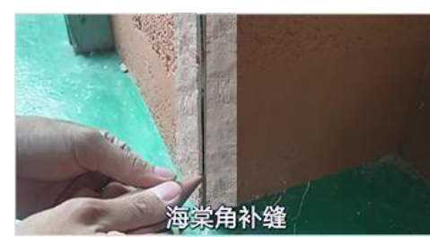
8. Fill the external corners with caulk
