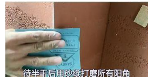
10. Grind the edges and corners
