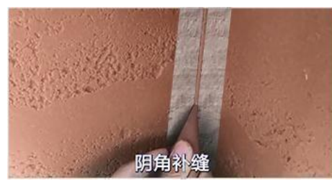
7. Fill the internal corners with caulk
