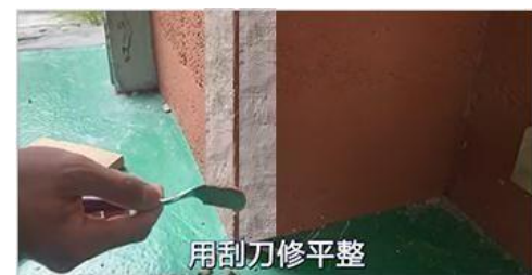
9. Use a scraper to smooth the caulk
