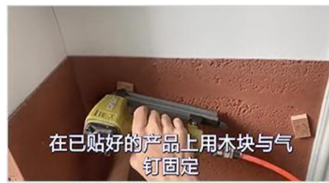
3. Fit it with air nails
